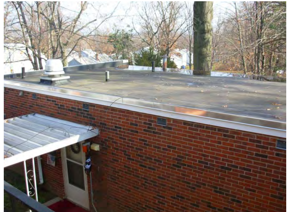
4. View of roof and canopy, note ponding
